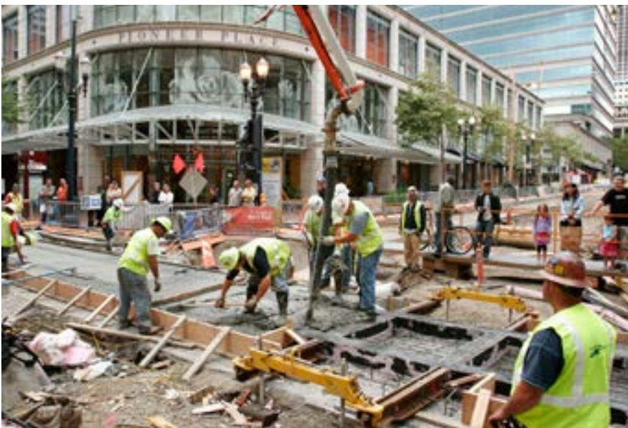
TriMet worked closely with contractors to speed construction. Crews worked double shifts in three to four block segments for up to eight weeks at a time.
