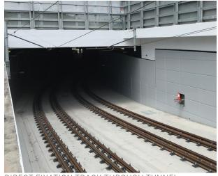
DIRECT FIXATION TRACK THROUGH TUNNEL IMAGE SOURCE: ZGF
