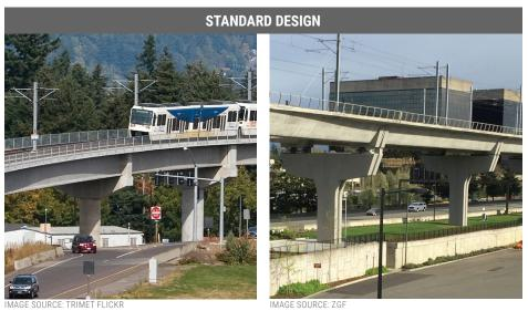
TYPICAL CONCRETE COLUMNS AND GUIDEWAY STRUCTURE
