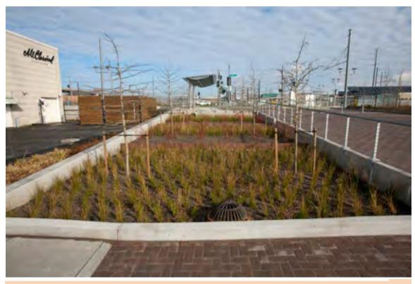
This large bioswale next to the OMSI/Southeast Water Avenue Station captures and filters stormwater diverted from the deck of Tilikum Crossing.
