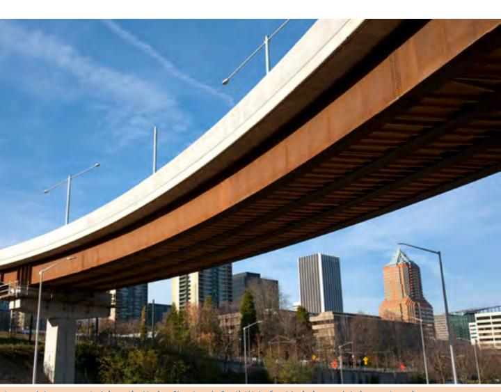
Low-maintenance materials on the Harbor Structure in South Waterfront include unpainted concrete and weathered steel. The steel girders were fabricated in Tigard, Ore.
